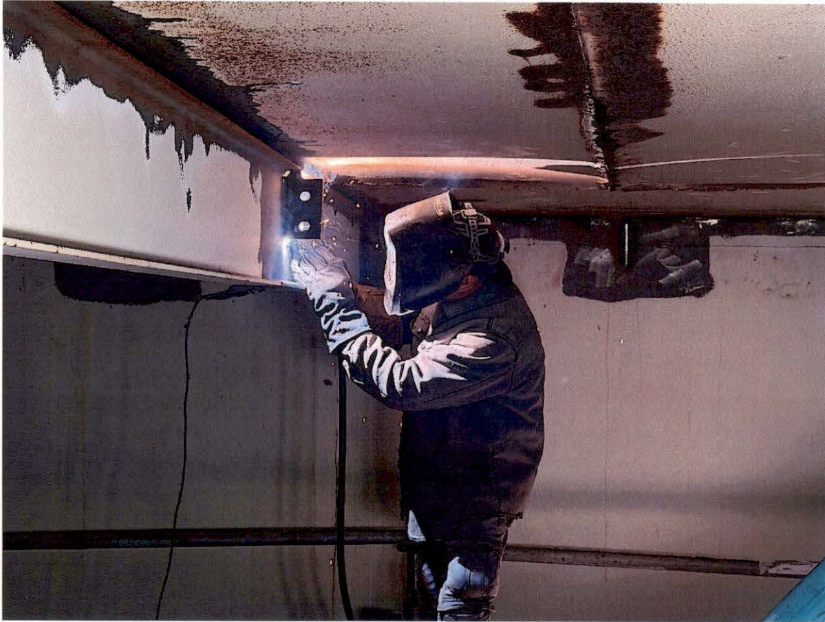
December 3, 2025 – Welding connection plate to the existing rafter.
