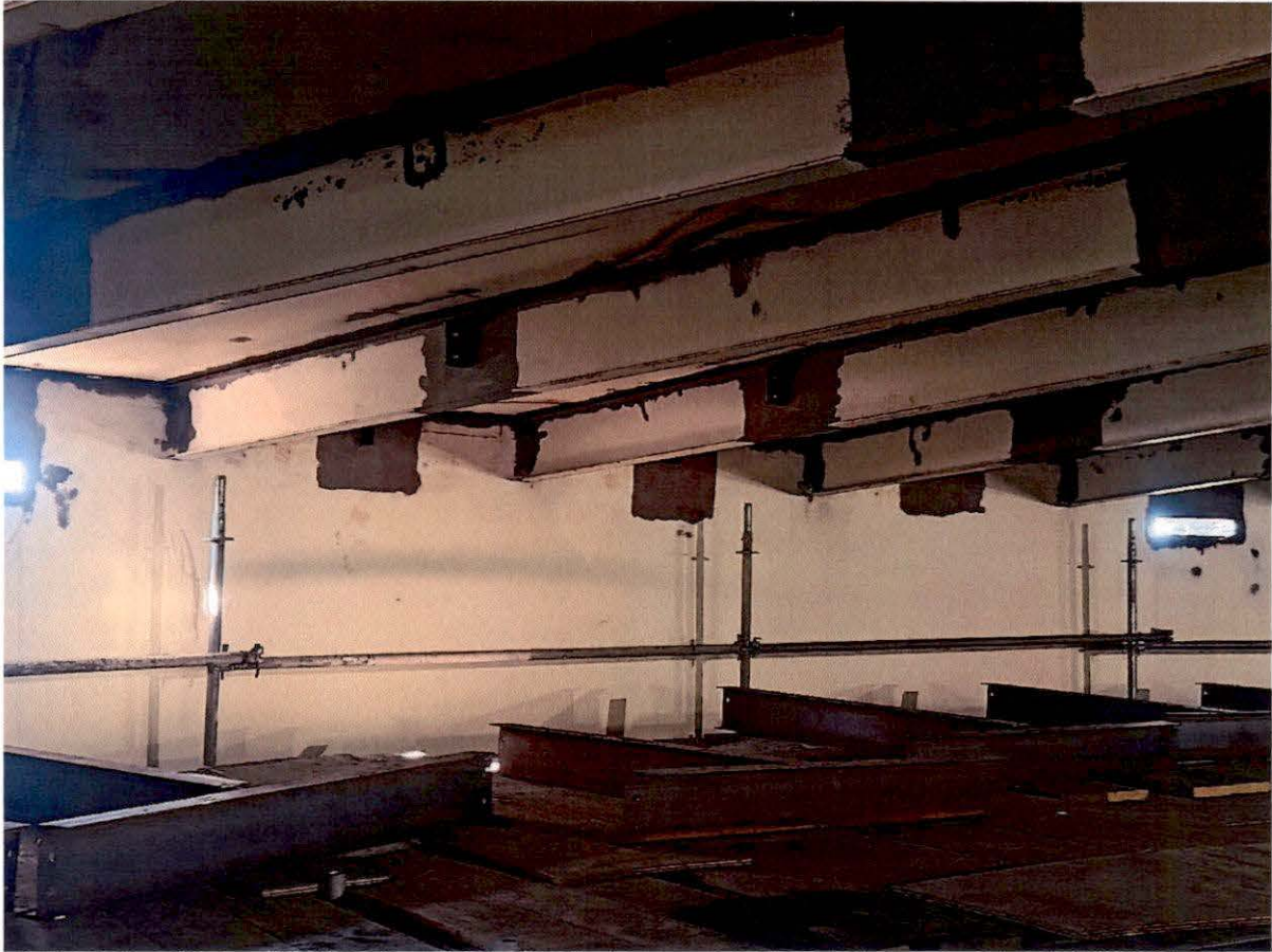
November 26, 2025 – View of new rafter assemblies (resting on scaffolding dance floor) waiting to be installed to the existing roof structure.
