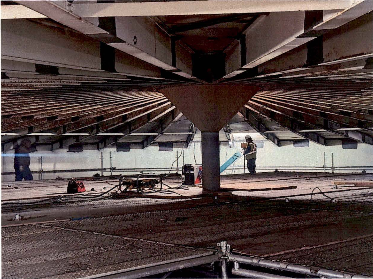
November 18, 2025 – View of rafters showing sandblasted areas where new welding and or new rafters will be installed.
